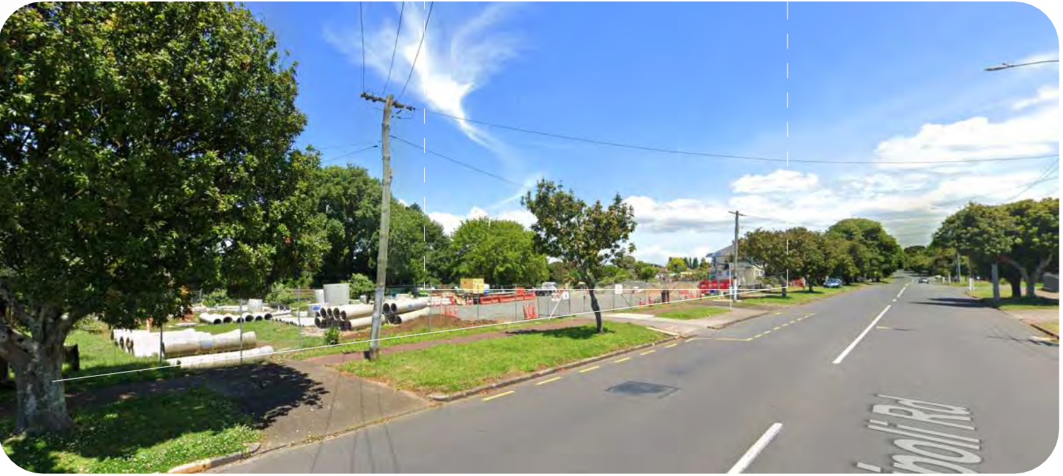
V3: The site frontage along Tripoli Road looking south, large titoki street trees line Tripoli Road
